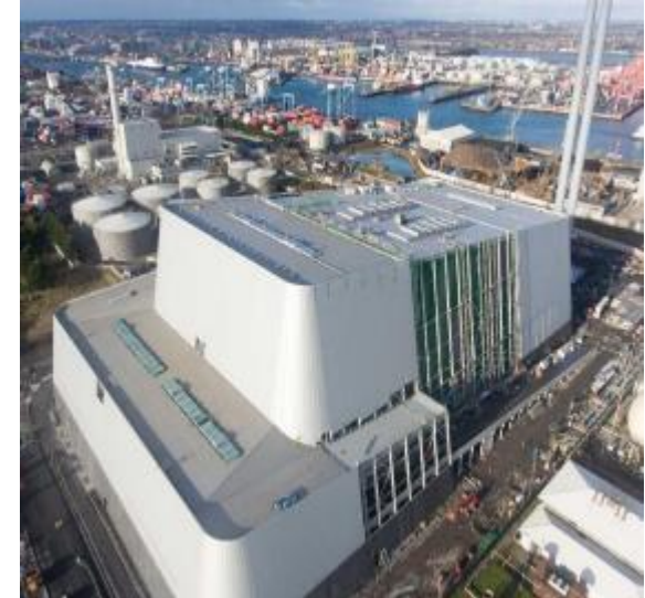
Dublin, Ireland – Covanta Energy
